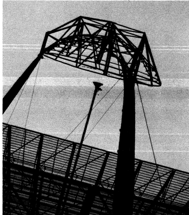
Close-up of the feed dipole. The dipole is covered with a polyethylene bag to keep rain water out of the assembly. The feed tower is guyed by use of a slip-ring collar, visible as the bulge half-way down the feed-tower. Since this photo was taken, a reflecting element has been added to the feed dipole, giving a cardioid feed pattern.
